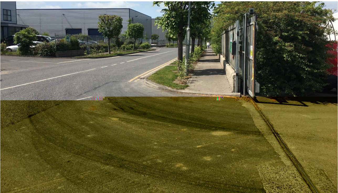
Figure 7-7: Grants Drive / Enva Site Entrance
